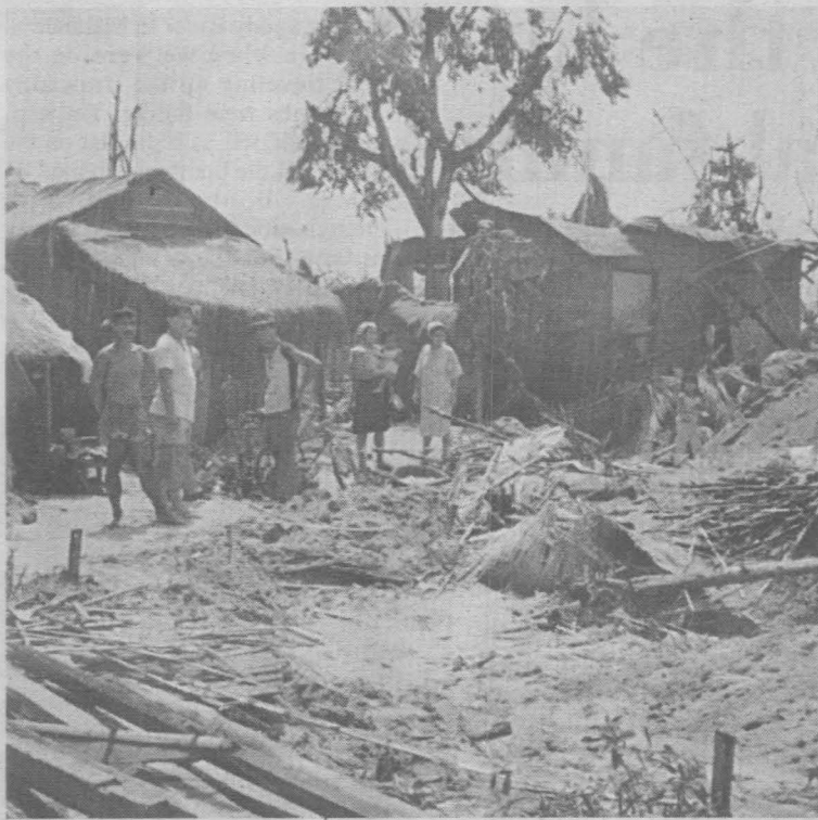
HOME SPARED —The nipa hut in which Moises Bangit, a member in San Felipe, Zambales, lives (hut at extreme left) was spared, while other huts collapsed under the weight of ash. [Photo by Conrado Cabrera]
