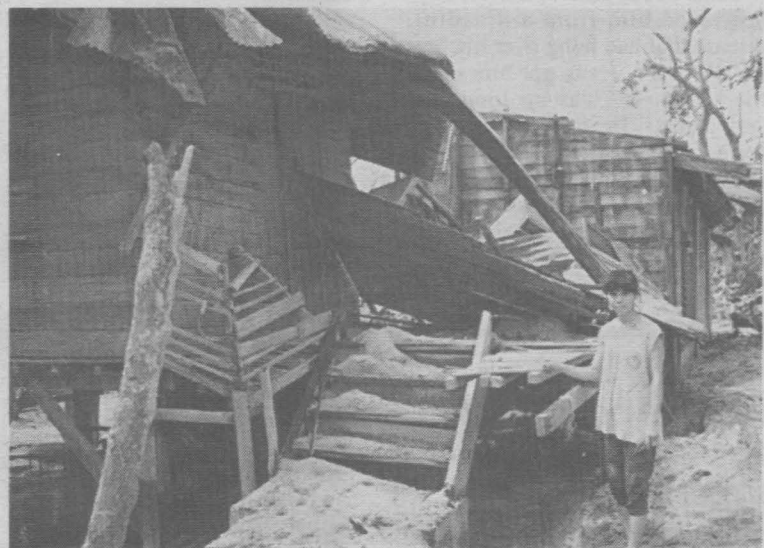
HOME IN RUINS—The roof of Angie Ramos' home in San Fernando collapsed under the weight of volcanic ash and sand. [Photo by Bill Sidney]
